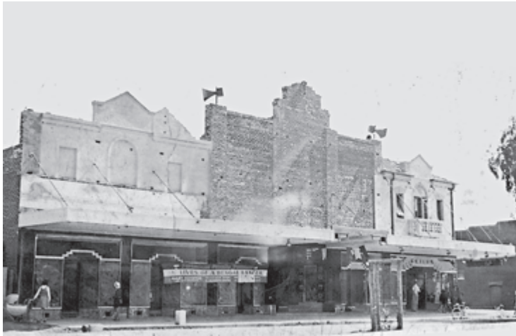
The Roxy Theatre with unfinished facade, April 1936. Between 1915 and 1963, Greeks operated more than 120 cinemas in some 57 country towns across the length and breadth of New South Wales.
